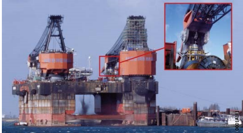
Figure 1 Rope sheave bearings in the crane vessel Hermod
